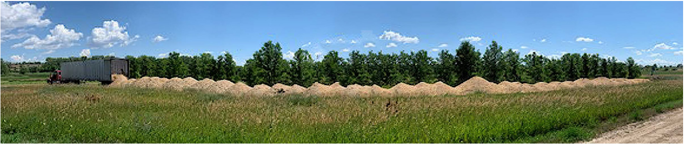
Pile Construction at Chatfield Farms, May 2020
