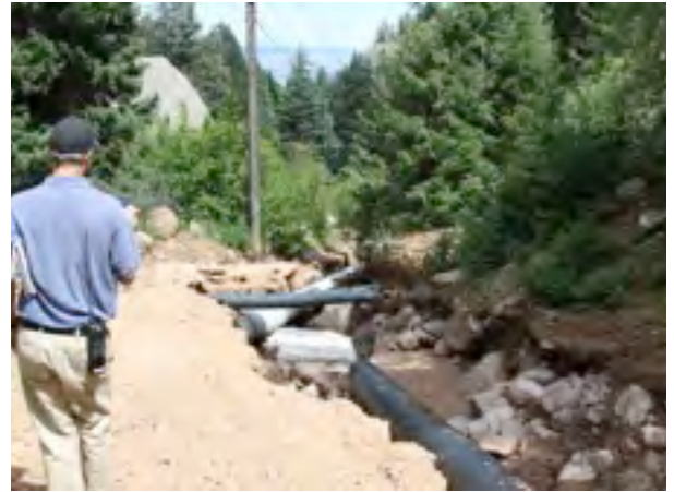
Figure 13 - Colorado Springs water line exposed by the July 30, 2012 storm event. Before the fire and the July 30th flood, this was a road. The pipelines carry water to Colorado Springs' main water plant. If this plant is lost the utility will not be able to supply water to 400,000 citizens and the U.S. Air Force Academy. They estimate a rebuild cost of around a billion dollars, and it would take years to rebuild.
