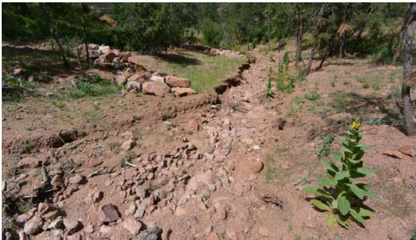
Failed, bendway weir
