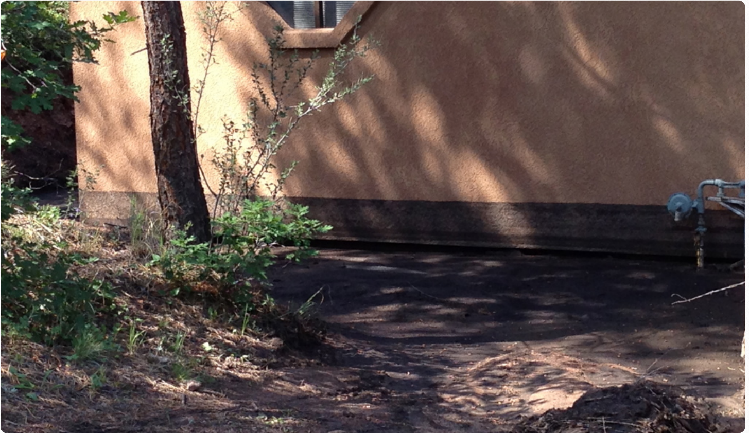
Mud flow line from a post-fire flood on a home in Cascade.
