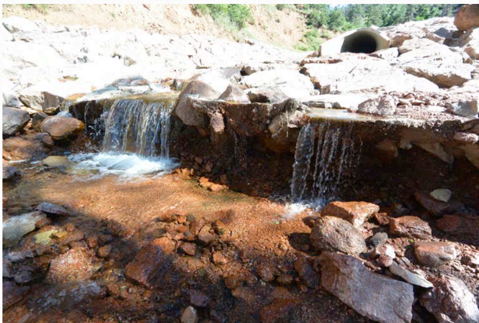
Grouted Rip Rap Channel functioning at risk as the toe begins to erode.
