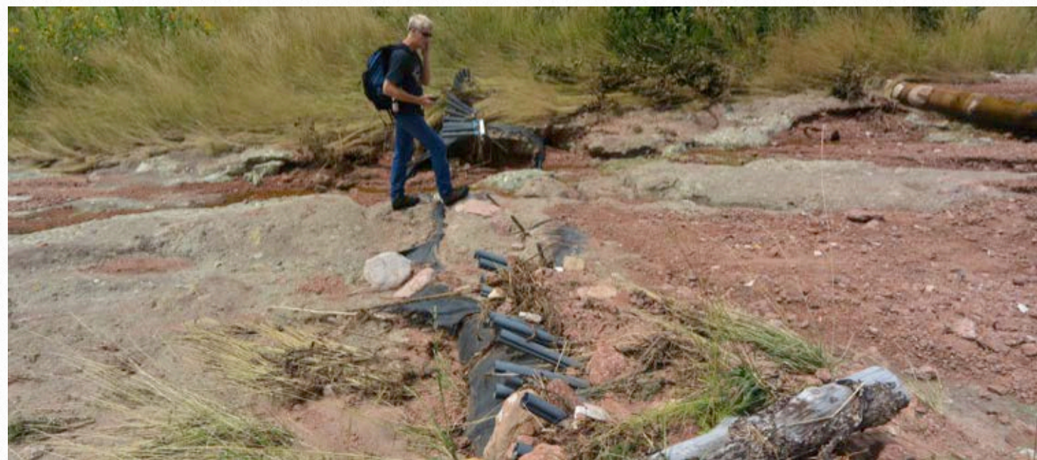
Damaged Whisker Sills: These were a new product recommended by a hydrologist, but they failed quickly.
