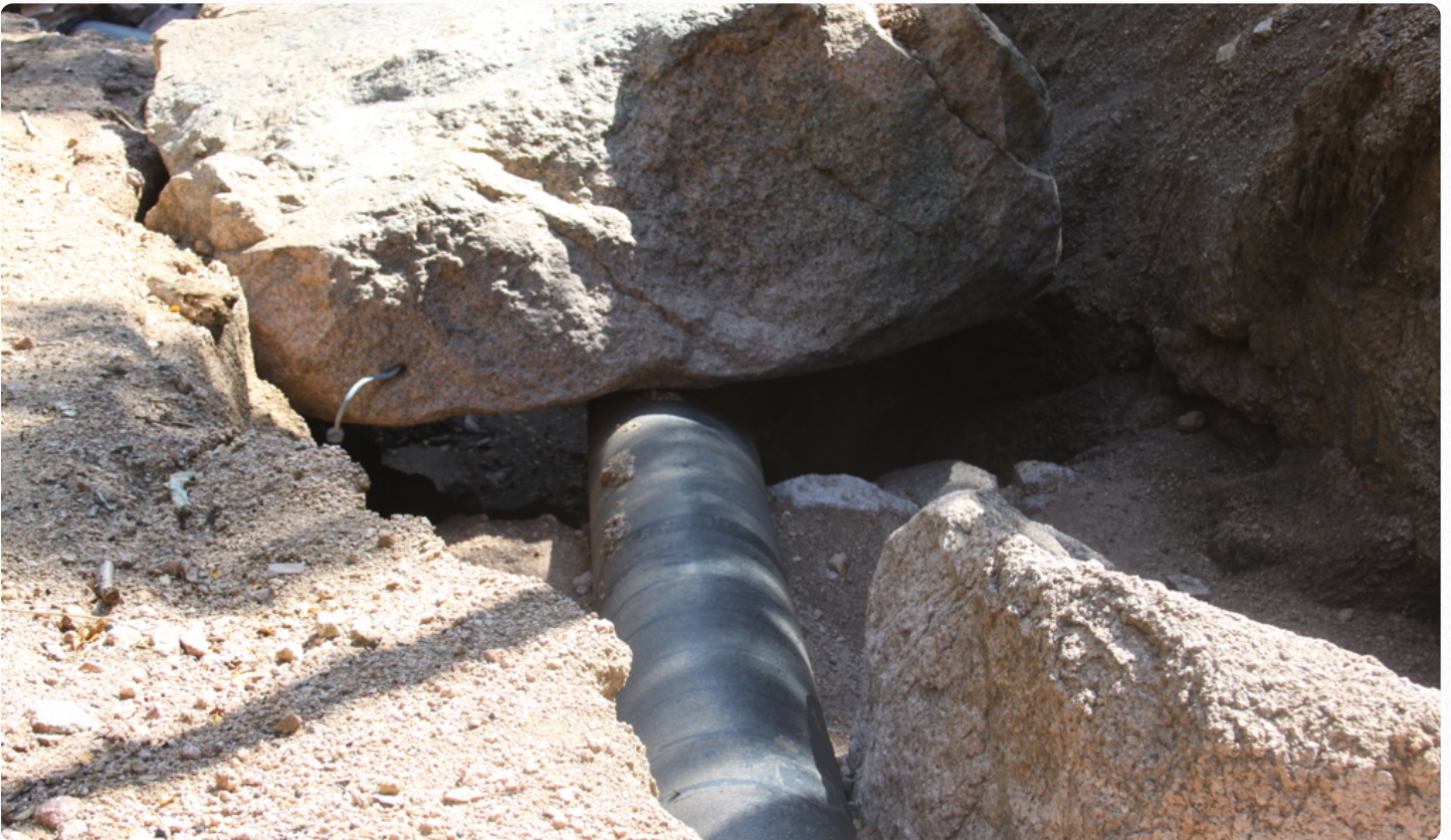
Post-fire flooding in 2012 exposed Colorado Springs Utility's backup pipeline from Rampart Reservoir, making it unsafe to run water through until repairs could be completed.
