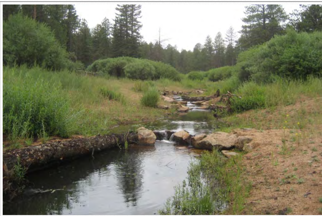
Channel reconstruction featuring new pool habitats formed by log J-Hook structures in Reach 2
