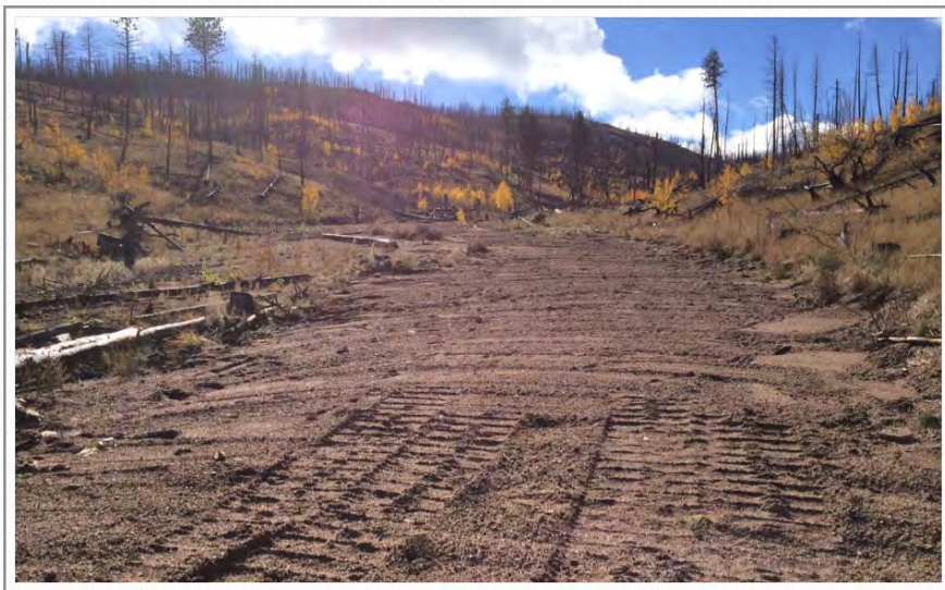
Filled down-cut channel in between the two sediment detention basins in Trail Creek Basin 60
