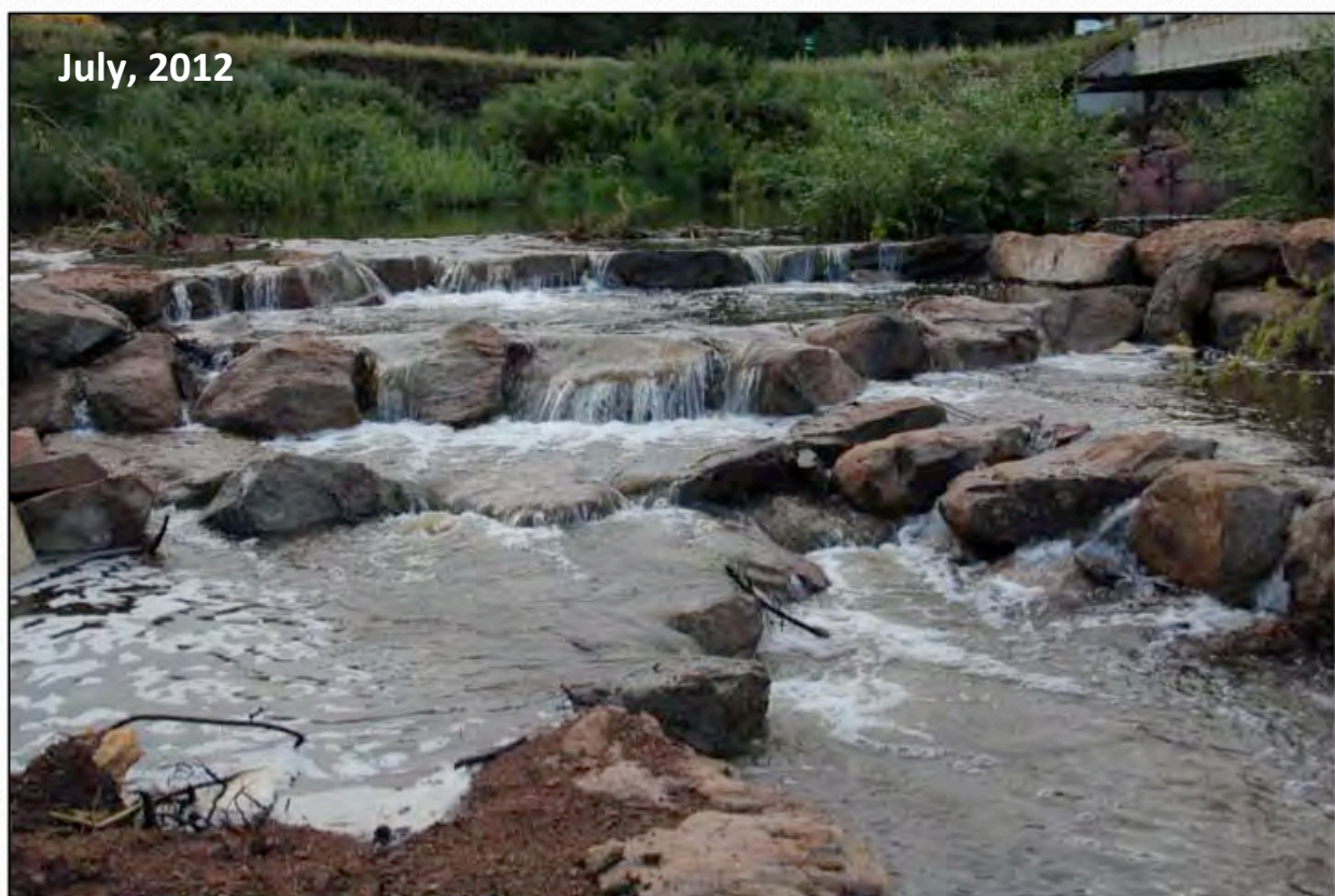
Before vs. After comparison below beaver dam on West Creek. A step-pool structure was used for fish migration, streambank erosion reduction, energy dissipation and grade control (constructed in July, 2012).
