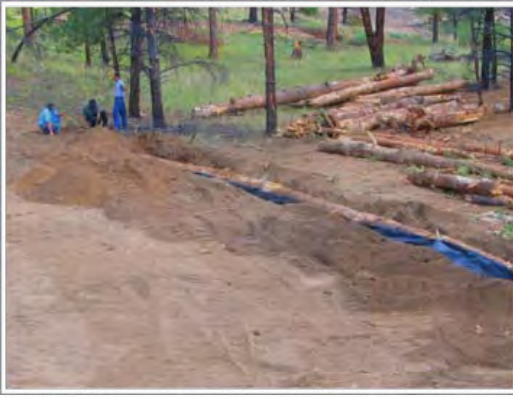
Sill logs installed with erosion control fabric help reestablish alluvial fans
