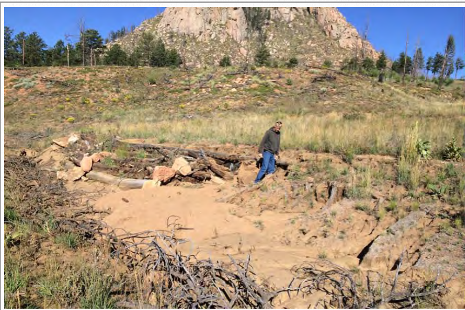
Partially filled sediment detention basin following August 2014 rain event
