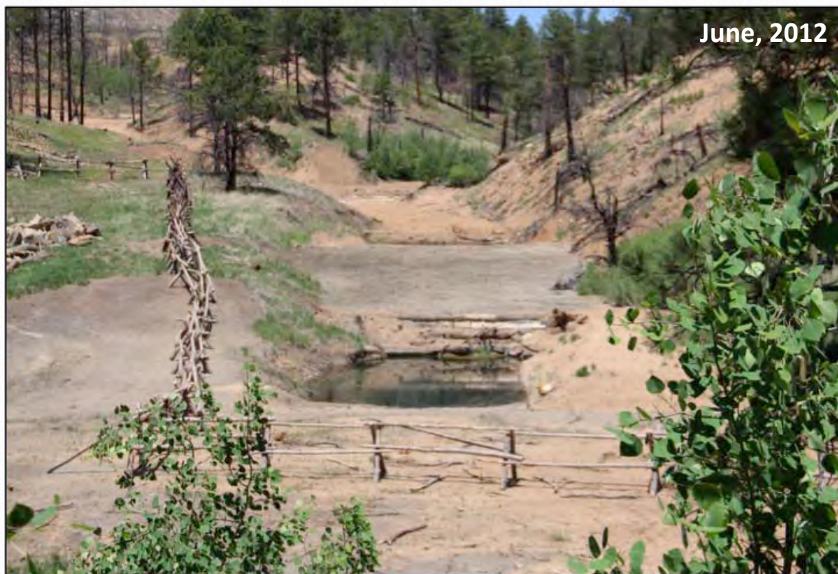
Headcut and incised F4b stream type at the mouth of Sub-watershed 6 showing Before vs. After comparison of sediment detention basin and braided, D4 stream type on raised surface constructed in November 2011.
