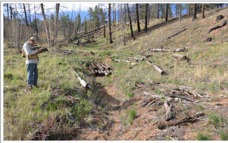
Layered log head cut stabilization structure in a small channel along the right edge of the fan
