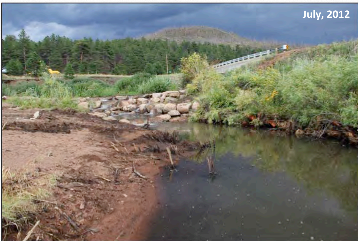
Before vs. After comparison of reach downstream of bridge on West Creek. Step-pool boulder structures were used to maintain beaver dam in place to prevent potential future headcut and breach. Toe wood was placed on bankfull bench in lateral scour pool created. Constructed in July, 2012.
