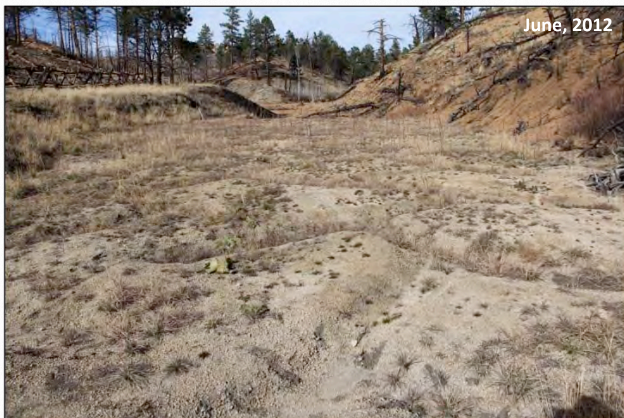
Before vs. After comparison of conversion of a F4b to a braided (D4) stream type as constructed in November, 2011 at the Trail Creek confluence of this tributary draining sub-watershed 6. Material from excavated sediment detention basins was used to raise bed elevation 5 feet and eliminate the gully with convergence/divergence, multiple channels constructed to disperse flow energy and deposit sediment. A 2-year storm in 2002 produced no sediment transport or flows into Trail Creek as flood peaks were diminished and sediment was stored on the new surface and in the constructed basins.
