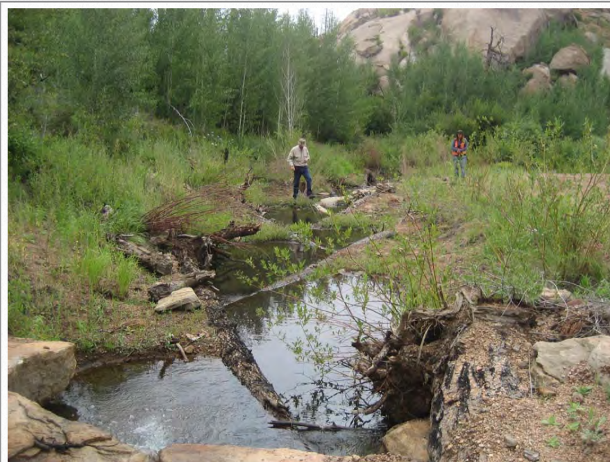
Channel reconstruction featuring “Rock & Roll” logs formed pools and new road alignment in Reach 4
