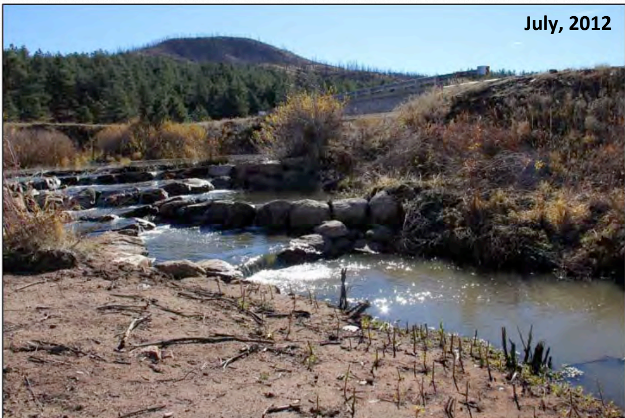
Before vs. After comparison of step-pool boulder structure on West Creek to prevent future breach of existing beaver dam. Note beaver dam immediately above invert of structure. A bankfull bench was constructed at the base of road fill. This reach was constructed in July, 2012.
