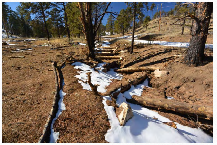
Log “Rock & Roll” structures on the main stem of Basin 6 below Stump Road - Basin 6 Fan #4 Site
