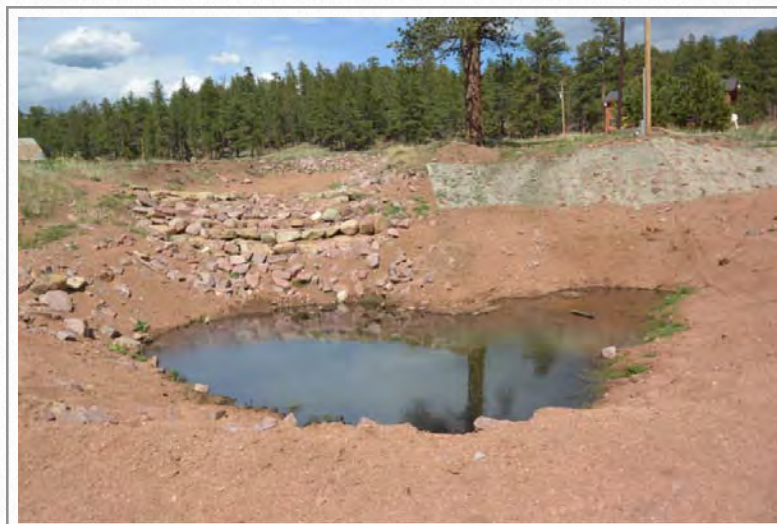
Sediment detention pond and drop structure at the downstream boundary of West Creek Ephemeral Draw #1
