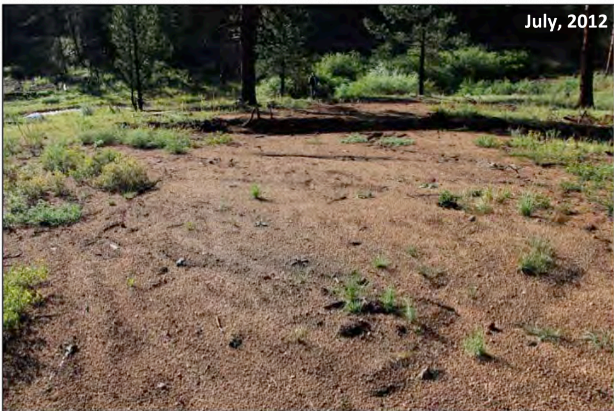
Before vs. After comparison of an unnamed tributary to Trail Creek showing a gully that was filled to restore alluvial fan function using excavated material from sediment detention basins as implemented in July, 2012. Stormflow runoff following a 1-inch+ storm was dispersed on the new alluvial fan surface as observed in the lower photograph. This reduced the high sediment supply from the gully and dispersed flood waters.
