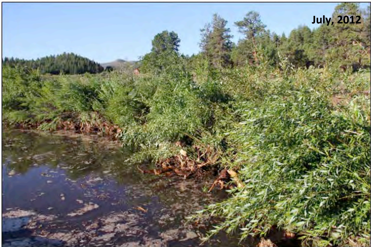
Before vs. After comparison of conversion of a braided (D4) to single-thread meandering (C4) stream type on West Creek showing the excavation and placement of toe wood with transplanted willow riparian vegetation as constructed in July, 2012. Beaver pond in background was reinforced for floodplain function and a raised water table.
