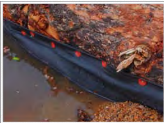
Erosion control fabric used for in-stream structures
