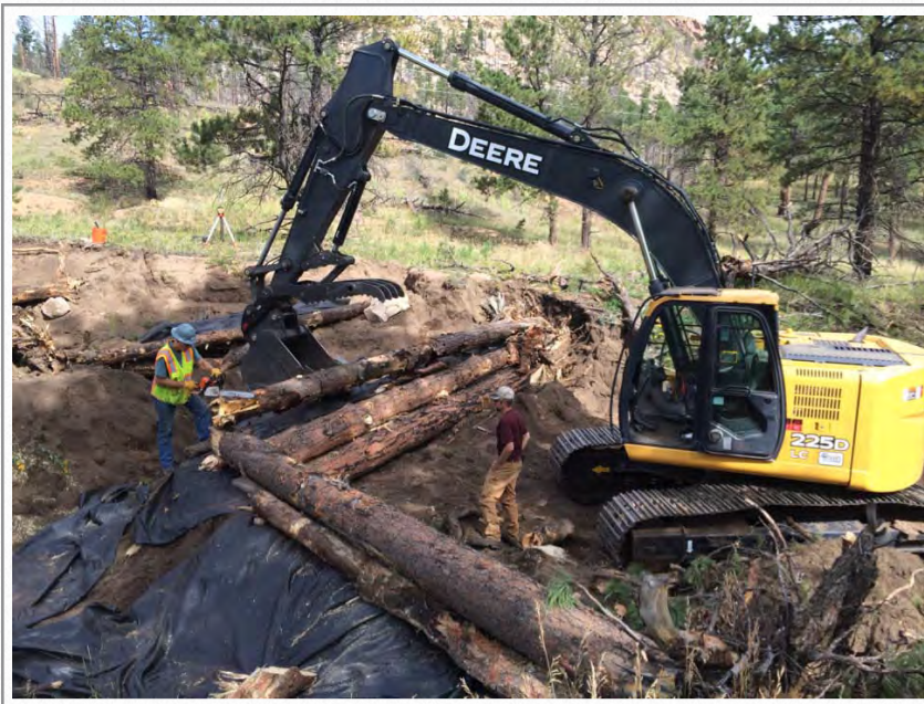
Constructing a log crib structure (2013 design) at the confluence of the two channels in Basin 6 Fan #4
