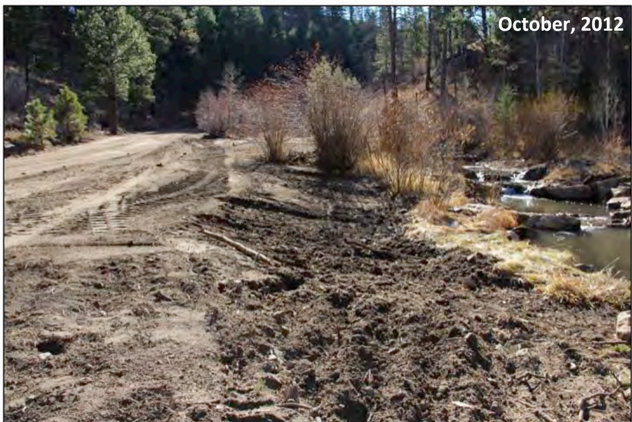
Before vs. After comparison of road and Trail Creek relocation that eliminated two ford crossings as constructed in October, 2012. Photographs are looking upstream.
