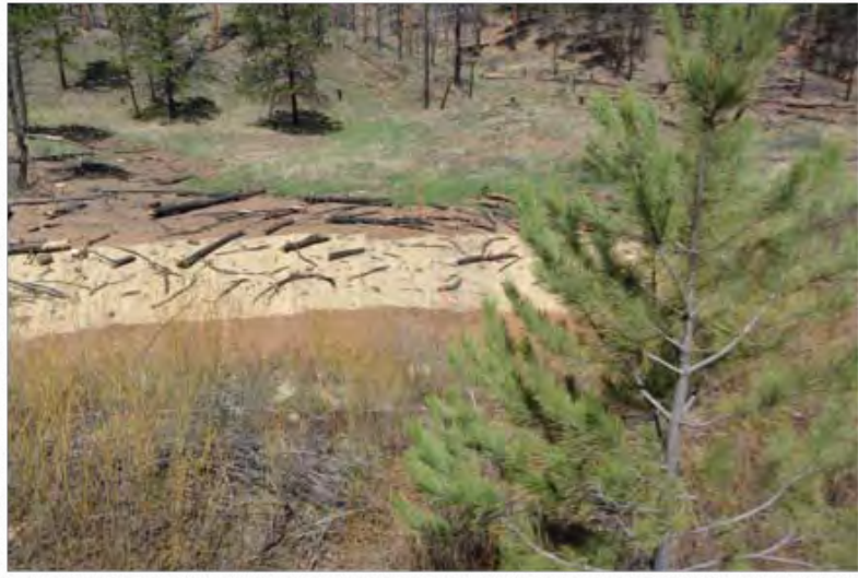
Treated fan toe and filled incised channel at Trail Creek Draw #7, adjacent to Reach 3
