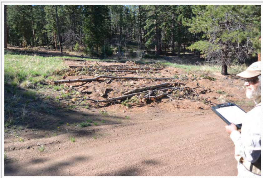
An F channel cutting through the fan in Basin #1 is filled, re-contoured, silled, and covered in slash.
