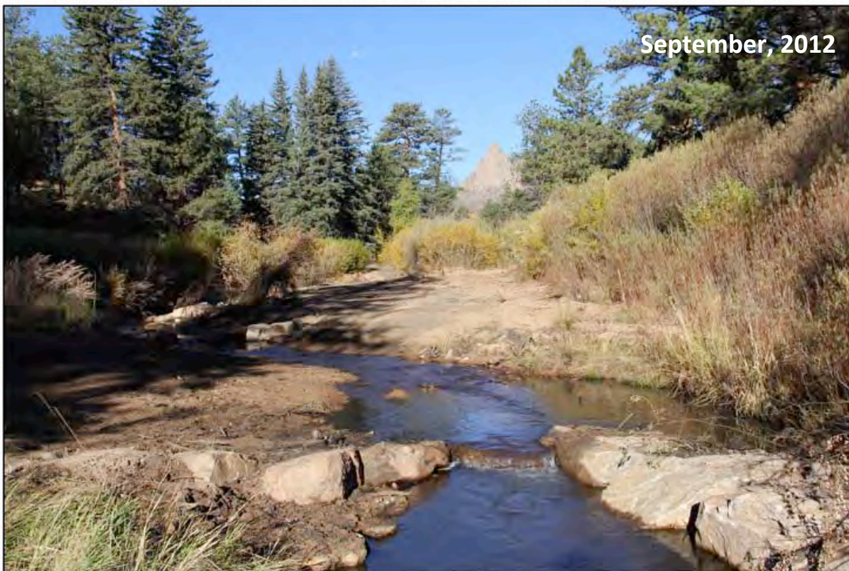
Before vs. After comparison of newly constructed, meandering C4 stream type (September, 2012).
