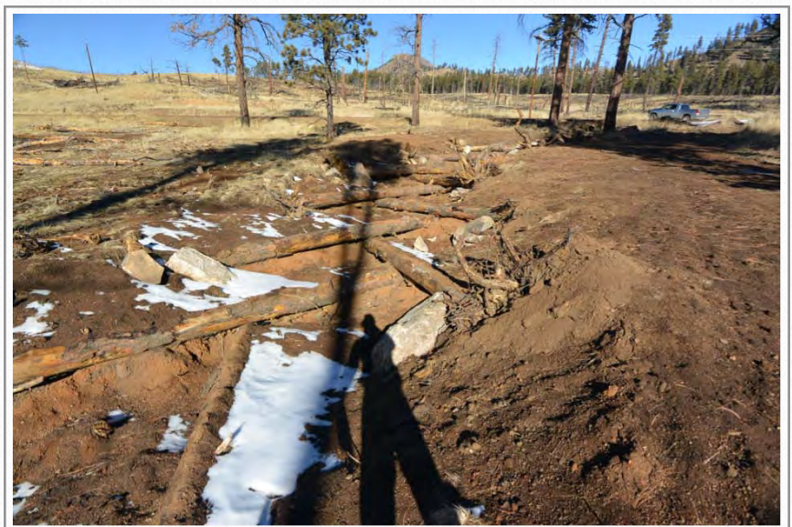
Log Rock & Roll structures on the stabilized channel through Basin 6 Fan #2
