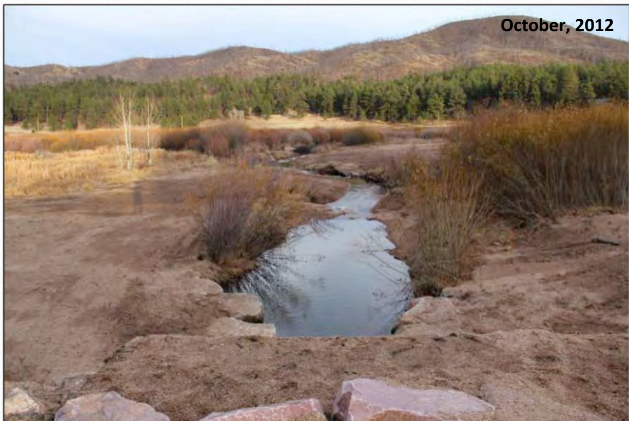
Before vs. After comparison of the downstream view of changes on Trail Creek at the West Creek road. The channel was converted from a braided (D4) to meandering (C4) stream type with removal of concrete barriers and re-establishment of floodplain as constructed in October, 2012. Aggrading channel was lowered 3 feet to match previous floodplain elevation behind the concrete barriers.
