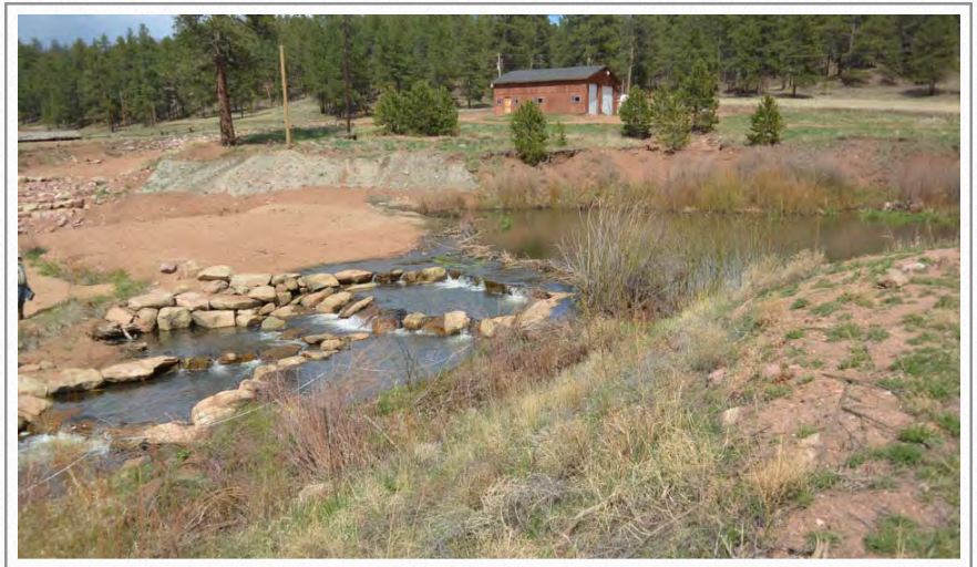
The boulder step pool structure at the top of West Creek Reach 1
