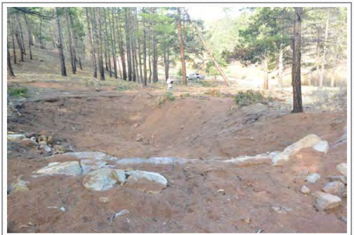
Sediment detention basin and restored alluvial fan at Trail Creek Basin 2Face3 work site.
