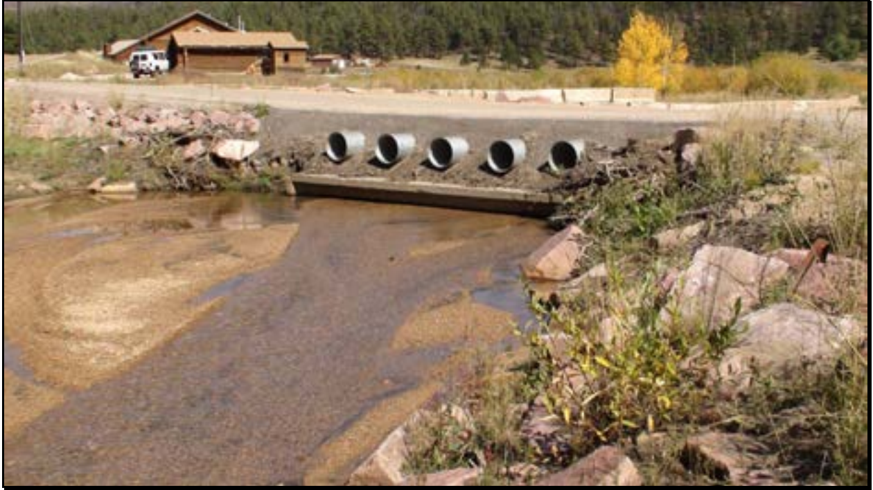
Figure 5. Aggradation due to poor road crossing indicating very high width depth ratio, D4 stream type in Trail Creek.
