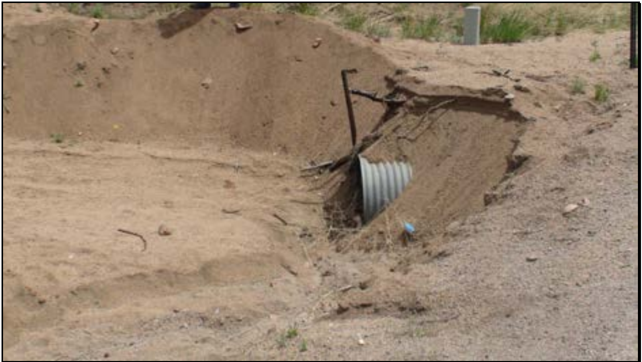
Figure 10. Sediment delivery from poor road drainage.
