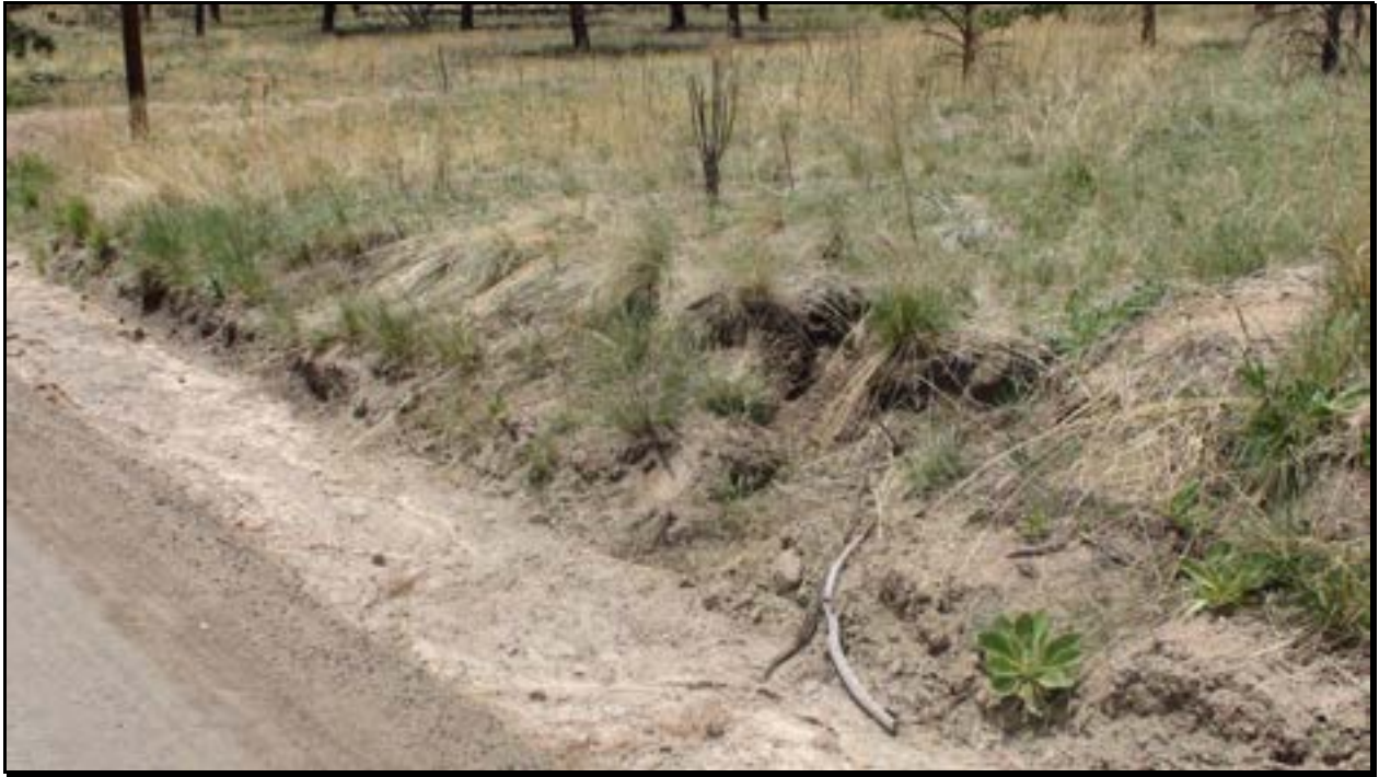
Figure 17. Sediment transported down the ditch line of a road in the Trail Creek Watershed.
