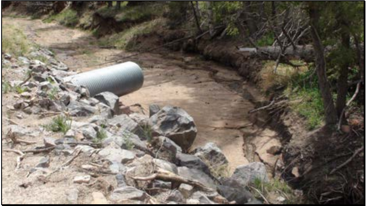
Figure 11. "Shotgun" culvert on tributary to Trail Creek converting a B4 to F4 stream type.
