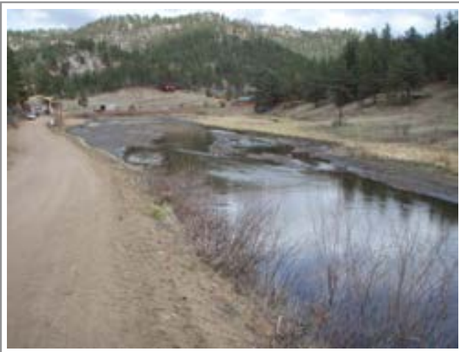
The channel behind the dam at Sportsmen's caused significant overwidening as seen above left. This threatened the road. Post project (above right), the channel is narrowed through backwater area of old dam, and has a meander bend.
