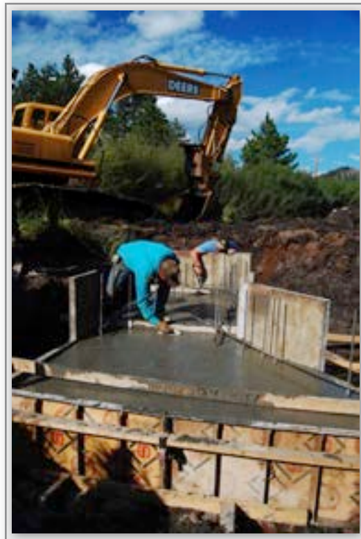
Construction of new headgate top two photos. New headgate at left.
