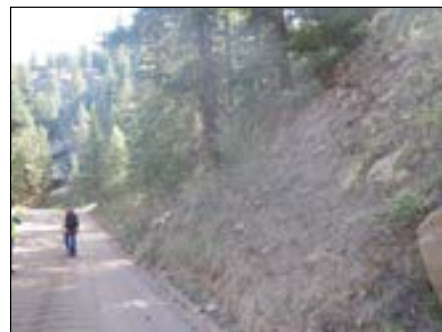
Photo 4 Typical Loose Cut Slope
