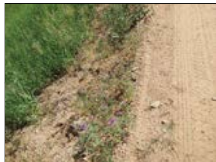
Photo 1 Shoulder with Loose Sediment
