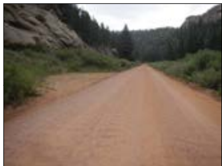
Photo 1 Typical Washboard Surface
