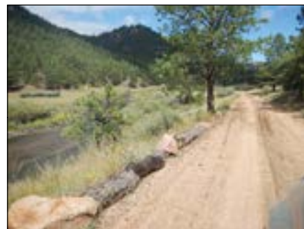
Photo 2 Roadside Erosion Protection
