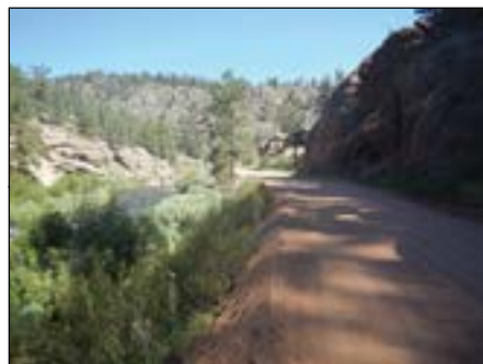
Photo 3 Typical Road Shoulder Drop
