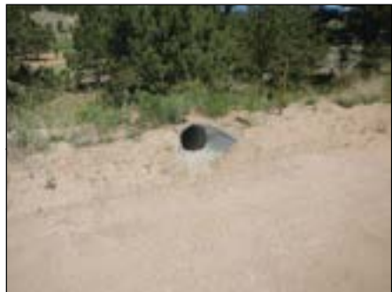
Photo 1 Culvert Rundown
