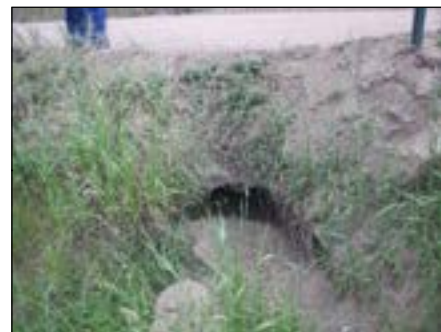
Photo 5 Culvert Blocked with Sediment
