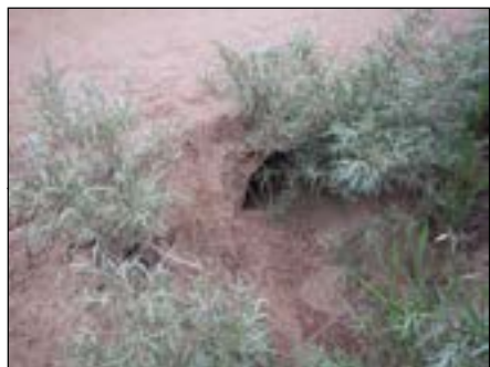
Photo 1 Culvert Blocked with Sediment
