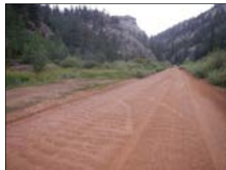
Photo 2 Typical Washboard Surface
