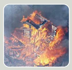
A home is fully engulfed during a fire in 2014. This house was not destroyed due to direct flame contact, but by the incursion of embers.
