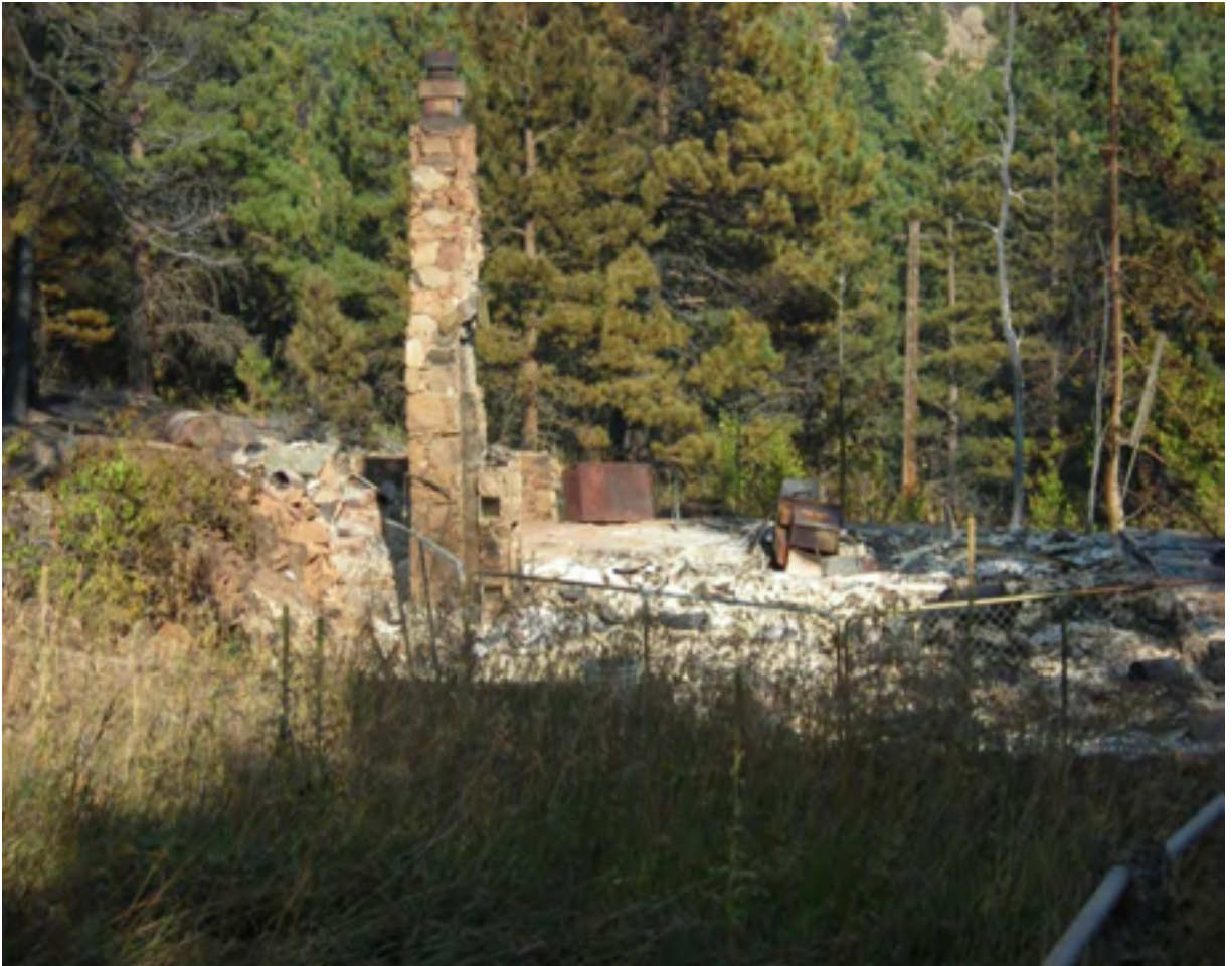
Figure 53. An example of total home destruction surrounded by unconsumed vegetation indicates ignitions associated with a low intensity exposure. The lack of available fire protection resulted in small ignitions sustaining and free burning to total destruction. Photo: Boulder County Sherriff.
