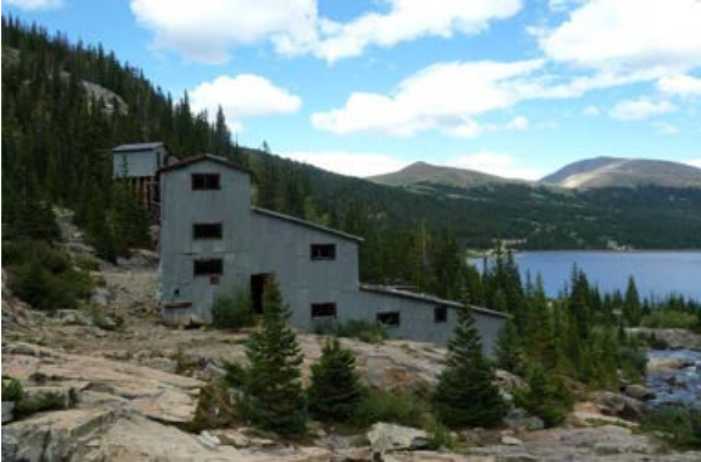
Photograph 18: Magnolia Mill, with Montgomery Reservoir in the background.
