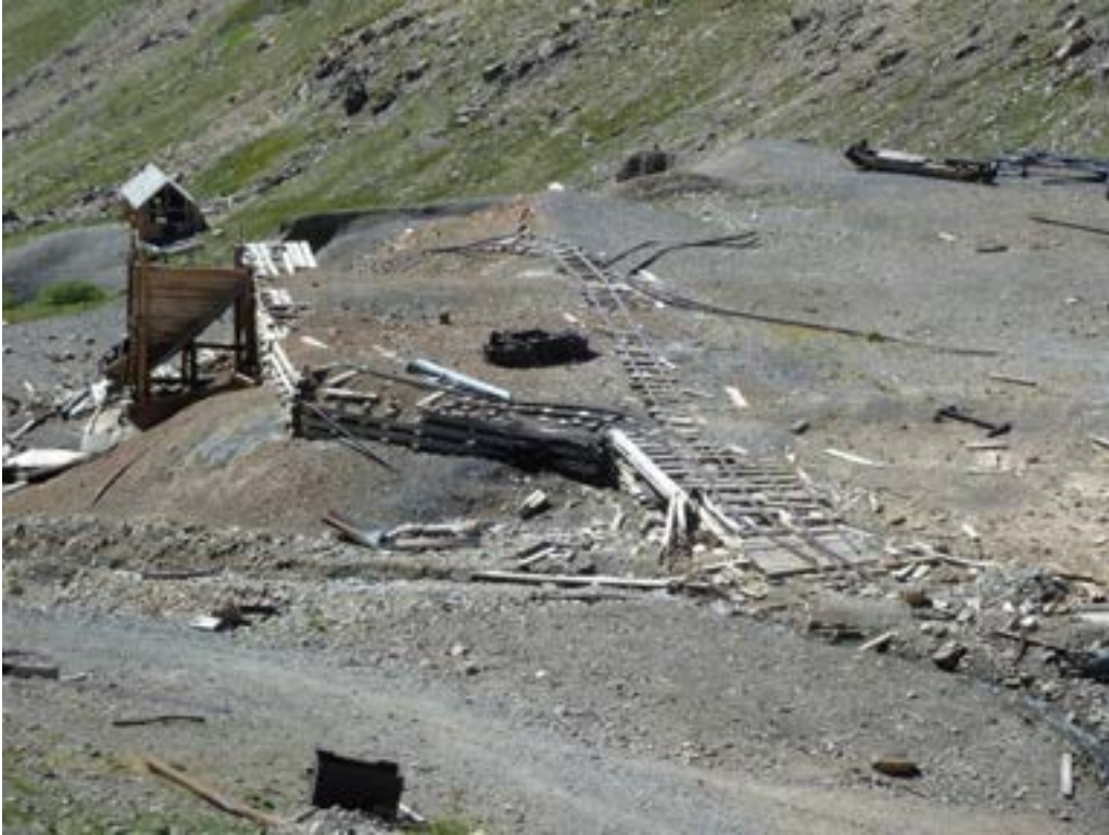
Photograph 31: Dauntless Mine complex.
