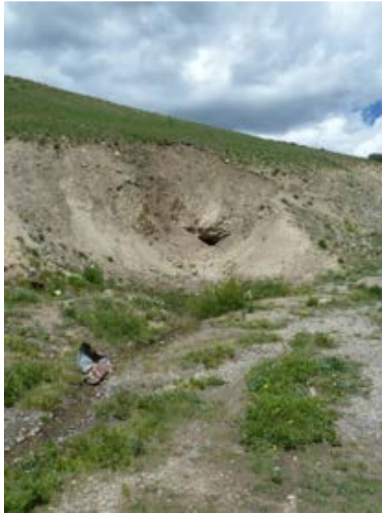
Photograph 28: Partially collapsed adit of the Ruby Mine, Weston Pass, South Fork of the Upper South Platte.
